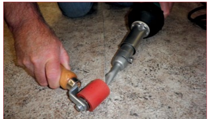
Welding with a hot-air gun provides a reliable, water-tight seal best obtained with the skilled techniques of professional installation.
