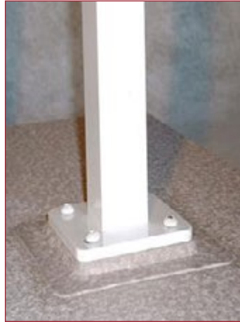
Raised base plate railing post detail.
