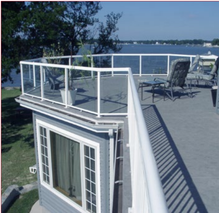
Roof deck by Duradek MidAtlantic
