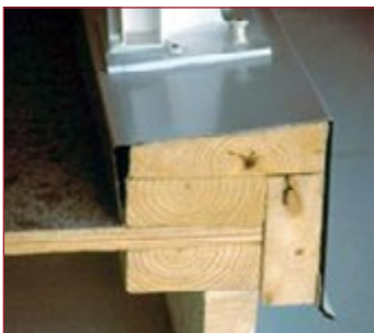
Cap Flashing on curb with 1 in 6 slope.
