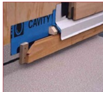
Sequencing details for flashing at inside perimeter.
