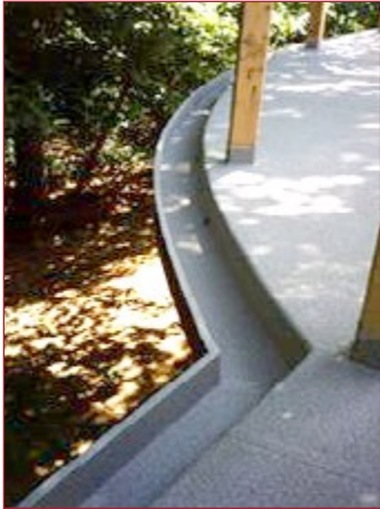
PVC coated gutter system with curves and corner details.
