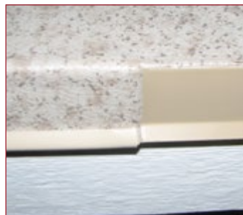
Outside Drip Edge Flashing: Option 1 - pvc clip over wrapped metal (left) Option 2 - pvc coated metal (right).
