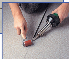
Trained applicators hot-air weld the overlapped seams for impenetrable protection.
