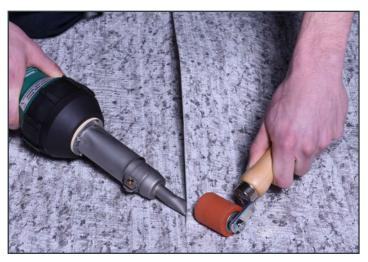
To allow for a strong, hot-air-welded seam, adjacent membranes should overlap by a minimum of 19mm (0.75 in.). It is important to remember proper fusing cannot take place when the back of the overlapping piece of PVC has been glued. Seam strength and integrity should be checked every few feet—if the seam comes apart, the welding is incomplete and must be redone.
