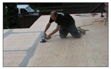
PVC deck membranes should not be applied directly to treated structural deck panels. Additives used in the various factory-applied treatments have caused 'backup' staining in the past. When pressuretreated plywood is required for deck construction, this author recommends an overlay with the aforementioned recommended plywood.
