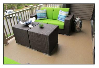
While waterproofing is the most significant attribute of a PVC membrane, appearance is also important. Vinyl products come in a wide variety of patterns, colors, and textures geared to diverse needs and budgets that can create complimentary or contrasting borders.
