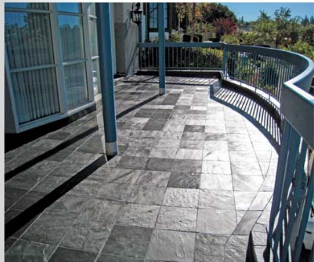
Finished tile deck, using Duradek Ultra Tiledek as the waterproof membrane.
