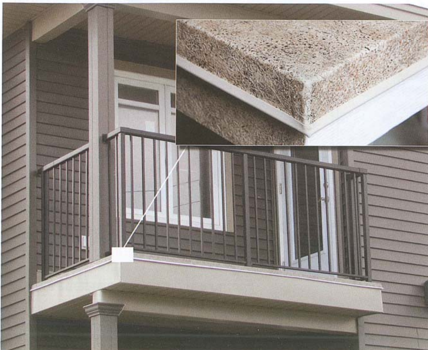
Check the flashing where the deck and house meet.
