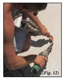
In either case, we make the joint between the deck and the collar watertight by welding the collar to the deck. Where we have to slit the corner to bend around the post, we weld on small corner patches. We use a similar welded patch at outside corners along the perimeter of the deck or where the deck meets the house wall. At inside corners, we use a "pig's-ear" fold for a neat, finished look.
