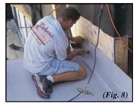
**Figure 8.** On the job shown here, Duradek was used as through-wall flashing for brick veneer cladding. The membrane covers the brick below and runs up the house wall and into the door opening. The remaining courses of brick were laid directly on the membrane, which directs any water trapped behind the brick onto the deck.
