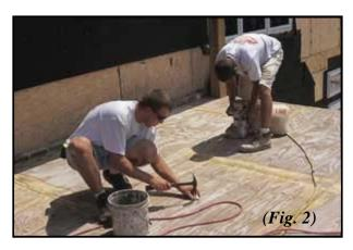
The first step is to fix any imperfections in the deck sheathing. Ideally, the GC will glue and screw the sheathing to the joists, countersinking the screw heads, but we can also work with plywood that has been nailed or stapled in place. First, we knock down the edges of the plywood joints and butt seams with a grinder, floor drum sander or edger using a light-grit paper (see Figure 2). Often, the sanding is enough to remove any dew or light surface moisture as well.
