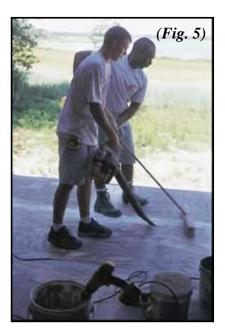
**Figures 4 and 5.** The crew smoothes the dried patching compound using a light-grit paper in a palm sander (above left). A once-over with a broom and a leaf blower clears the deck of any wood chips, roofing granules, and other debris that could get trapped under the membrane (above right).
