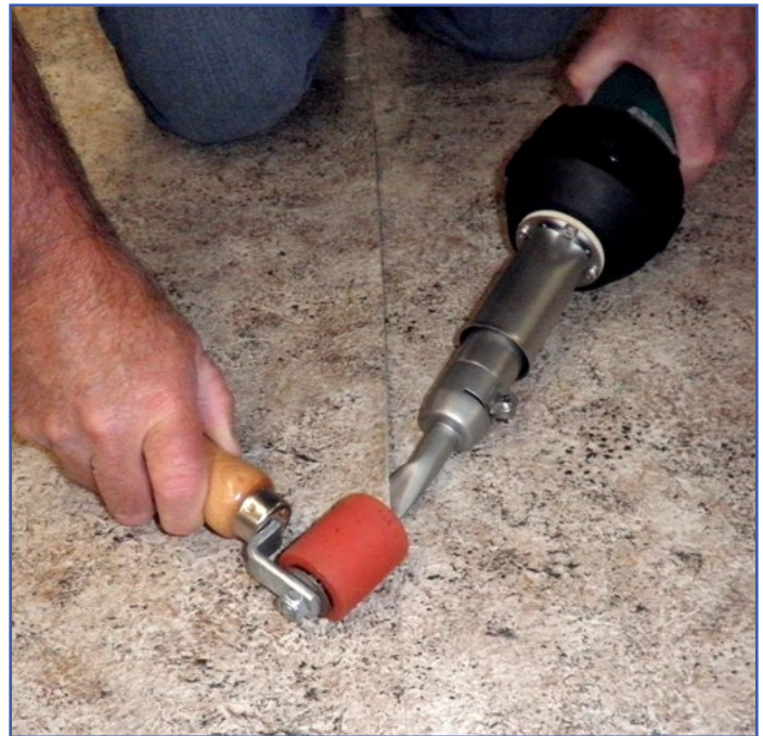
Duradek' heat welded seam fuses the vinyl sheets together, creating a completely water tight seal.
