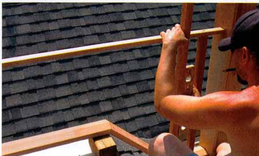
Figure 7. A simple painted cedar railing finishes the deck (left). Balusters are attached with screws through a rail insert at the top (below). A V-shaped notch at the base of each baluster (bottom) matches the beveled top of the shoe rail.
