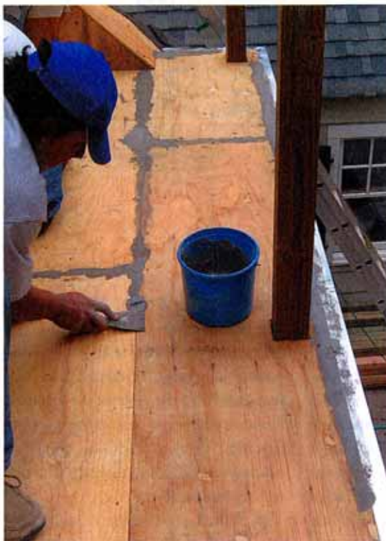
Figure 2. After installing the metal perimeter drip edge, the Duradek installers patch joints, nail heads, and voids in the plywood deck with a silica-based floor filler (above), then sand the deck smooth (above right). Sealant fills the joint between the deck and wall sheathing, preventing the membrane from forming a water-collecting crease (right).
