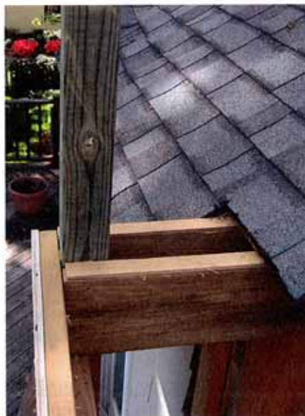
Figure 1. Tapered strips of framing lumber glued and screwed to the deck joists supply the necessary 2 percent slope for drainage (top). Four-by-four PT railing posts are bolted to the framing (right) before the plywood deck sheathing is installed (far right).
