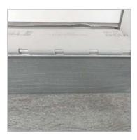
Step 7 The pre-flashed door threshold was finished by heat welding the vinyl sheets together, then covered with the composite trim.
