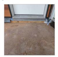
Step 2 The door threshold was pre-flashed with Duradek vinvl prior to cladding installation.
