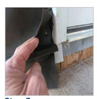
Step 3 The cladding was installed to an 4" clearance with access to the pre-strip moisture barrier behind pre-flashed moistured barrier overlap.
