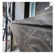
Step 1 Vapor Barrier/Building Paper was installed on exterior walls and on 2x4 metal-wrapped fascia.
