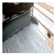
Step 8 A custom diverter was created for the outside corner of the deck edge to ensure surface moisture management.
