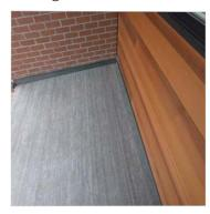
Step 10 Composite board was installed as a trim to complete the roof deck with a attractive finish.
