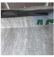
Step 6 Vinyl was applied to the substrate and up the walls behind a pre-strip vapor barrier.
