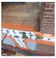
Step 5 The fascia was covered in pre-finished flashing with pre-strip vapor barrier.
