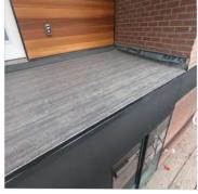
Step 9 The flashing was fastened to the fascia. Then fascia was wrapped in metal for a clean, contemporary finish.
