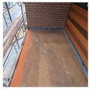
Step 4 The deck substrate preparation was completed with a 2% slope.
