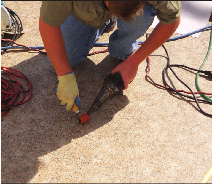
Heat-welded polyvinyl chloride (PVC) roof seams create a watertight seal.
