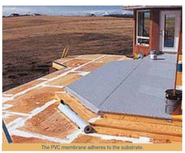
For a roof deck membrane installation featuring PVC and coated metal elements, the PVC membrane is heat-welded to a PVC-coated flashing that provides a drip edge at the outside perimeter of the deck surface. The PVC membrane is heat-welded to a PVC-coated scupper box, which provides drainage, and to a PVC-coated overflow drain that also provides drainage for trapped or curbed decks.
