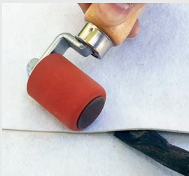
Fig 2: 1½" triple-welded seam
