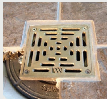
Fig 3: Cast Drain with Nickel-Bronze Strainer
