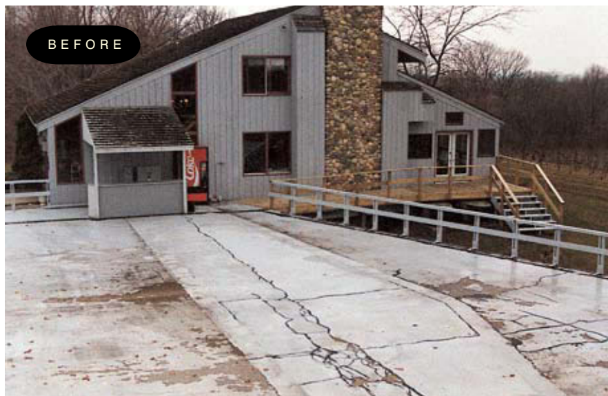
LEAKING, UNSIGHTLY ROOF OVER WINERY
